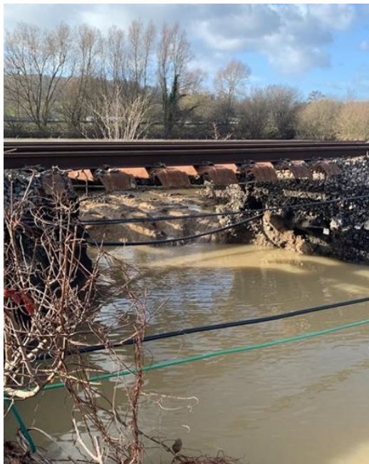
Photos of some of the washouts. Photographs: Network Rail.
