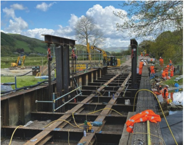
The lifting blocks with the chains attached.
