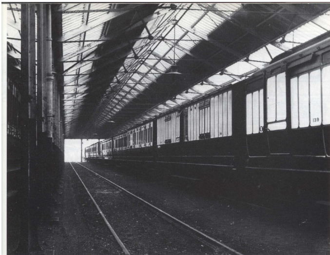
The interior of Carlisle carriage shed in 1907. Going out of picture to the right is 45ft bicycle van No.139. Next comes 45ft full brake No.94, followed by a 42ft x 8ft 6in lavatory composite to P53 or P57 and 42ft x 8ft lavatory composite to D158 with a coupe at the far end. Notice the light section bridge rail and fine grit ballast almost up to rail level. (Photo LGRP 7998)
