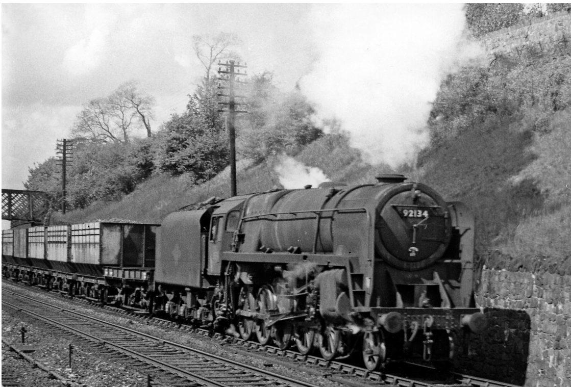
2.4.1 A BR Standard Class 9F with a train of unbraked mineral wagons on the Midland Main Line. Whilst the 9F was a very capable, fast and modern machine, its ability to move the traffic along quickly is being hampered here by the low speed necessary for operating unbraked freight trains. Generally this was no more than 25 mph.
